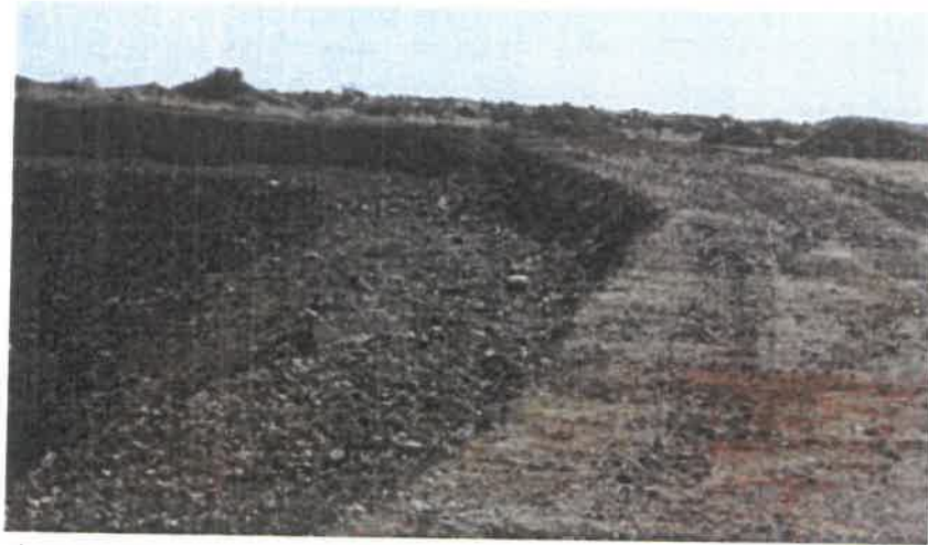
Photo 8: Typical perimeter safety bench during hard-rock quarry rehabilitation
