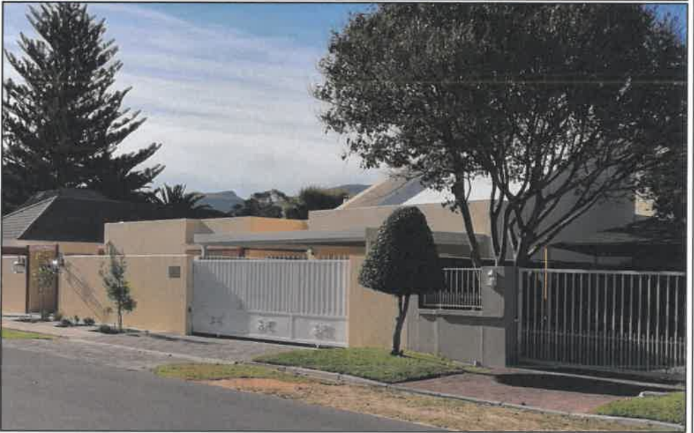
Figure 10: Photos of the existing carport
