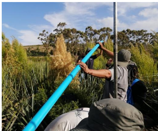
Monitoring wells being installed.
