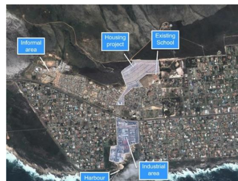
Figure 15: Kleinmond integrated housing development
