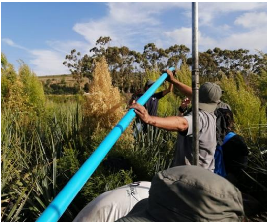
Monitoring wells being installed.
