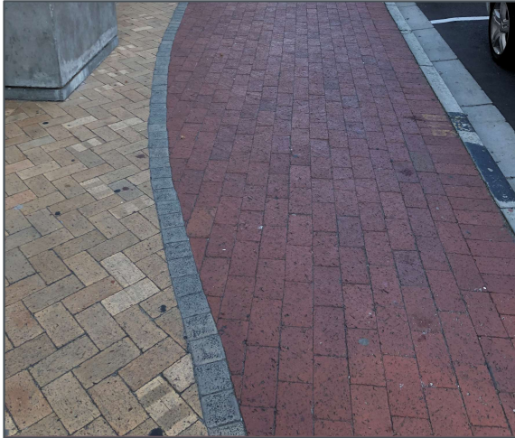
Unobstructed routes with clear line of sight destinations.
