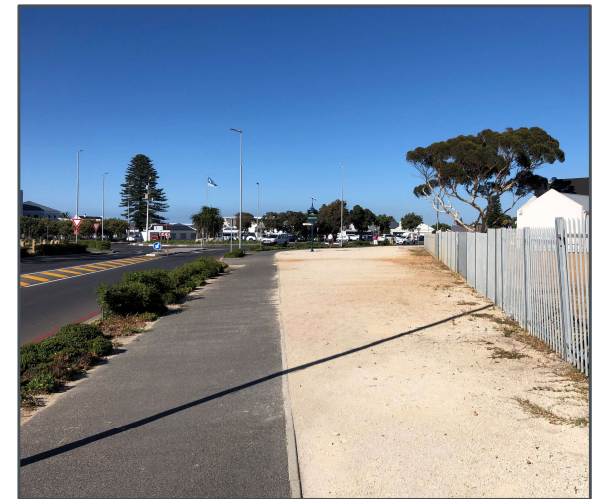
Separation of NMT from road by means of landscaping.
