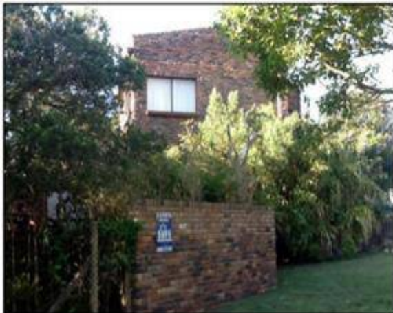
Fig 2 Corner west wall and north fence
