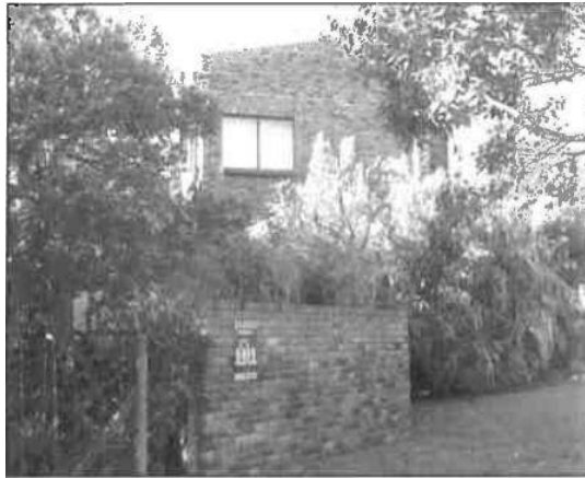
Fig 2 Corner west wall and north fence
