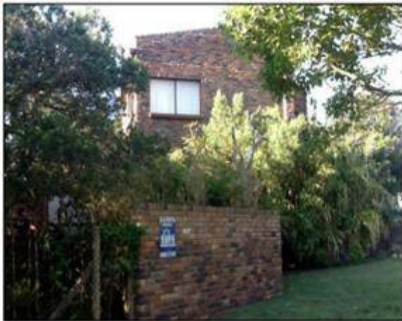
Fig 2 Corner west wall and north fence
