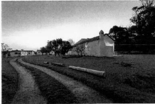
10. Existing access road to self-catering units
