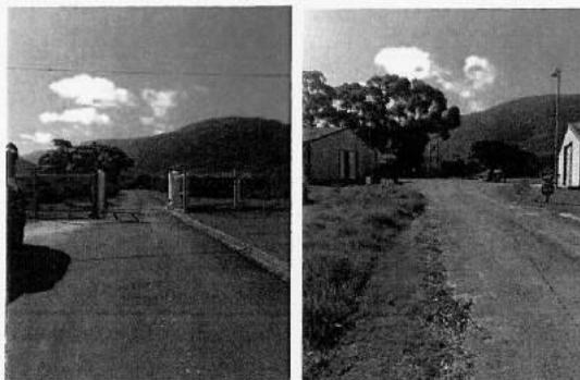
6. Existing access gate and tarred farm road
