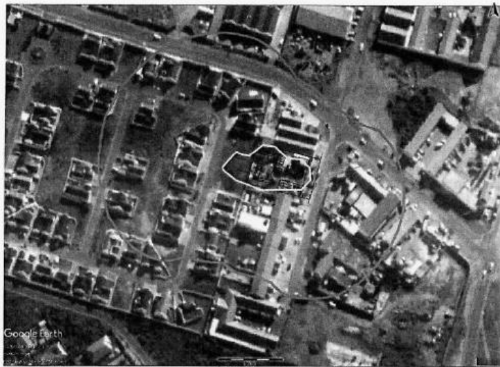
Individual Risk for the Proposed Installation
