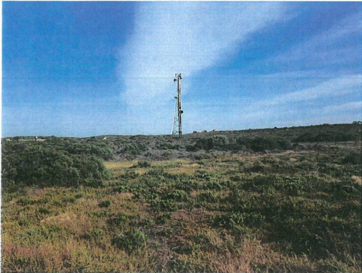
Figure 2: Visual Impression of a Lattice Mast.
