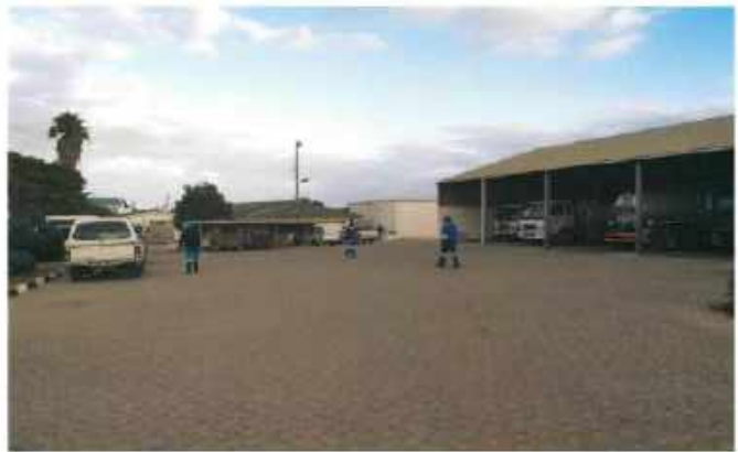
Upgrading of Municipal Workyard
