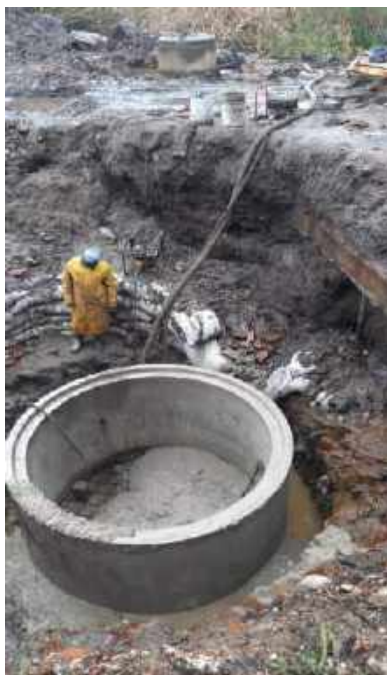
Left: Upgrade of the Kidbrooke Sewer Pipeline
