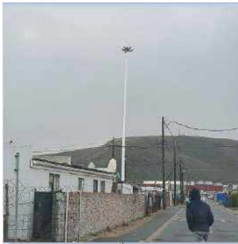
Installation of new high mast light in Zwelihle
