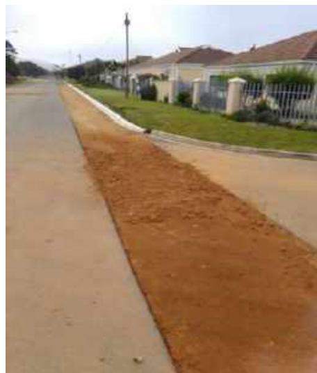
Extension of sewer network in Kleinmond
