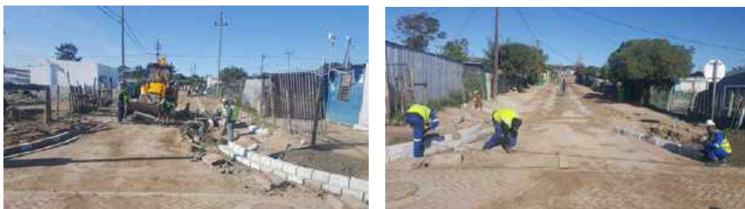
Rehabilitation Roads, Stanford Phase 2
