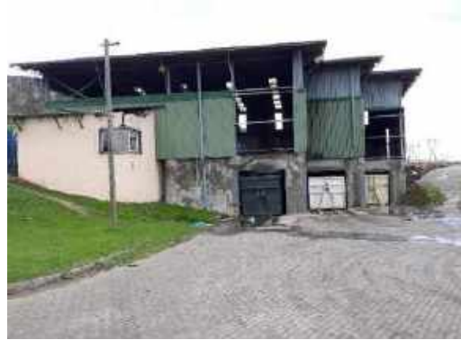
Kleinmond Transfer Station before repairs
