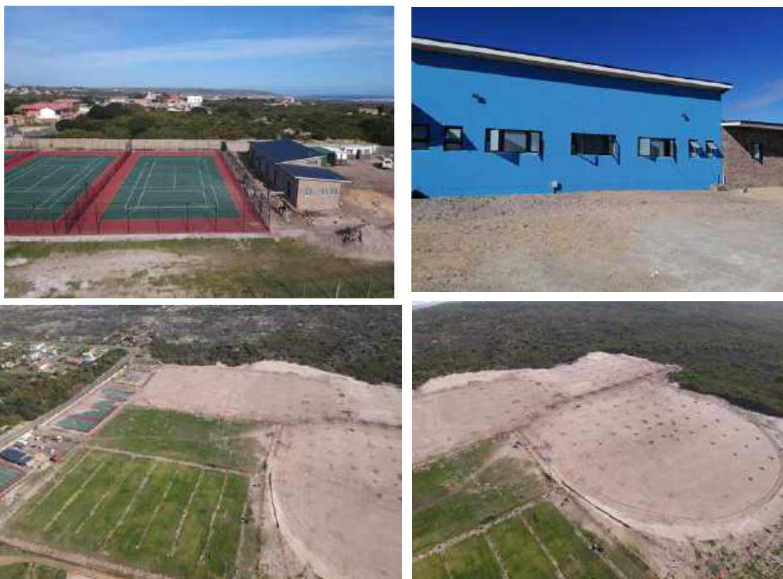
Phase 2 under construction- Hawston Upgrade Sport Grounds
