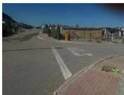
Sidewalks construction, Masakhane, Gansbaai
