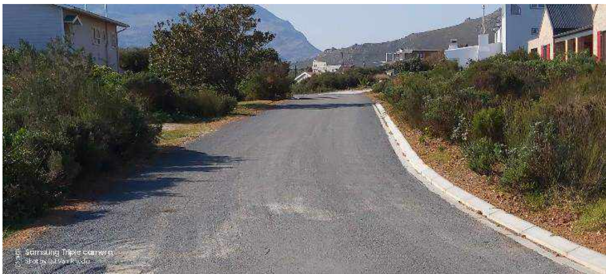
Dust Control of Vivian Road, Pringle Bay
