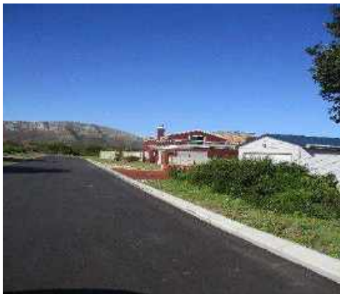
Stanfords Cove in De Kelders - installation of kerbs and paving on the sidewalk of a portion of Cove Street.
