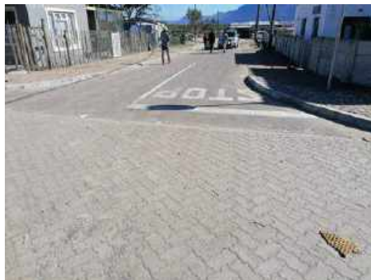
Stanford roads rehabilitation – Phase 2
