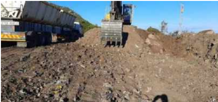
Removal of the old Hawston landfill to Karwyderskraal Landfill site
