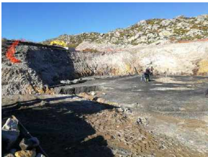
New reservoir being constructed at Pringle Bay.
