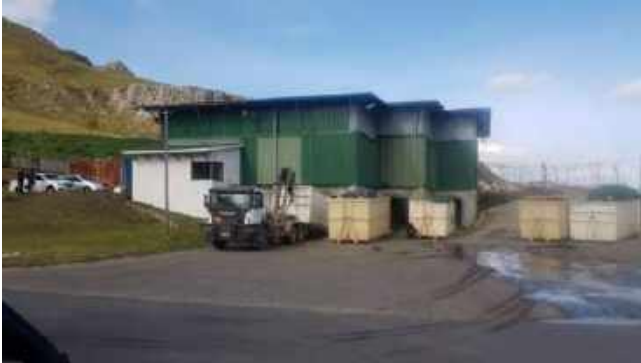
Kleinmond Transfer Station after repairs completed
