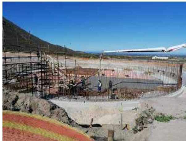
NEW 4ML RESERVOIR UNDER CONSTRUCTION
