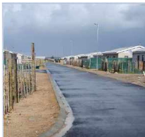
Electrification of Hawston Housing project in Hawston
