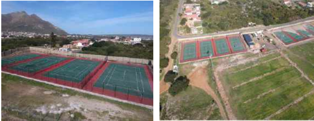
Phase 1 completed- Hawston new netball and tennis courts
