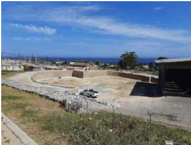
Repaired garden waste drop off area at the Kleinmond Transfer Station
