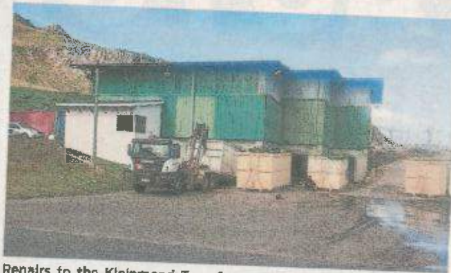
Repairs to the Kleinmond Transfer Station are almost done.
