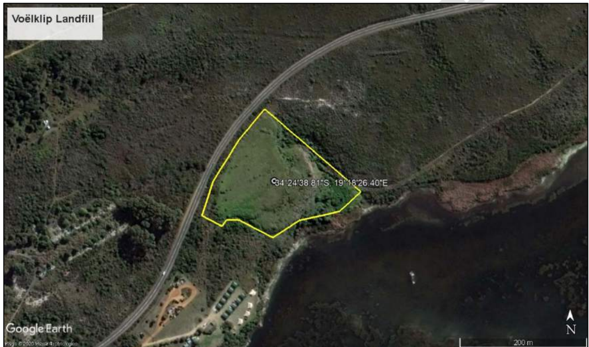
Figure 2-15: Voëklip Closed Disposal Site
