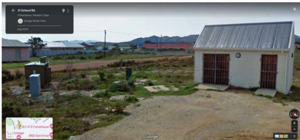
STREET VIEW OF PUMP STATION
