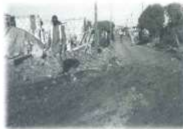
Roads under construction
