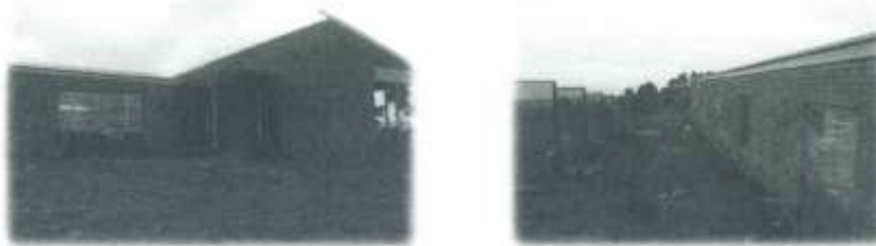
PMU Building Under Construction
