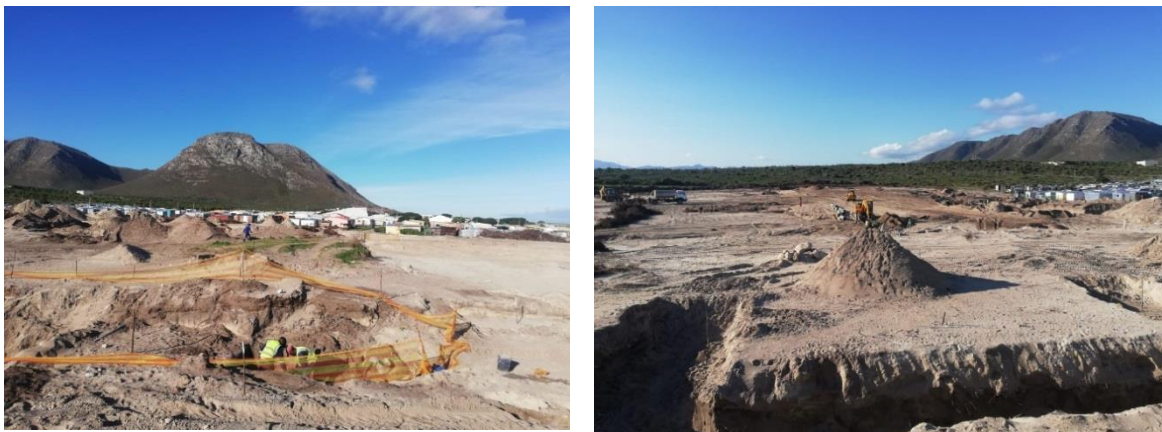
Masakhane IRDP project, Civil Works
