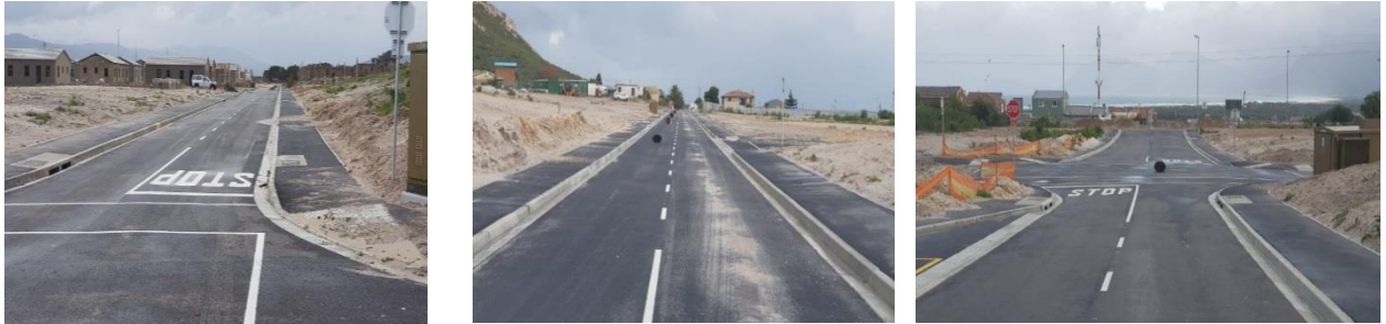
Hawston Housing project bus route – completed
