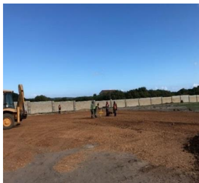
Phase 1 in progress- Hawston new netball and tennis courts
