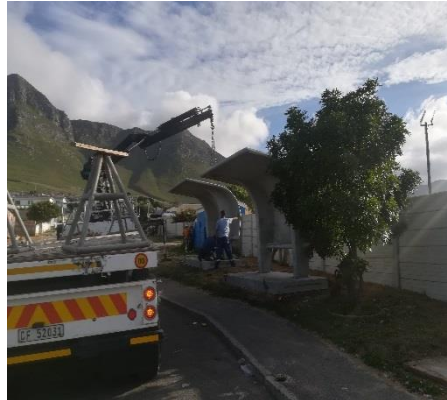
Erect concrete bus shelters in Protea road, Proteadorp
