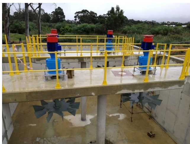
Upgrade of the Stanford Waste Water Treatment Works (WWTW)
