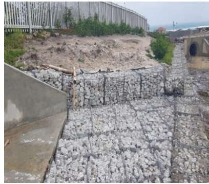
Hawston Housing project Bulk Storm water project completed
