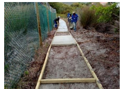
Concrete footpath and fencing (Heuningkloof footpath)
