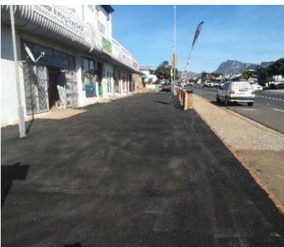
Resealing of asphalt sidewalk in Main Road Kleinmond
