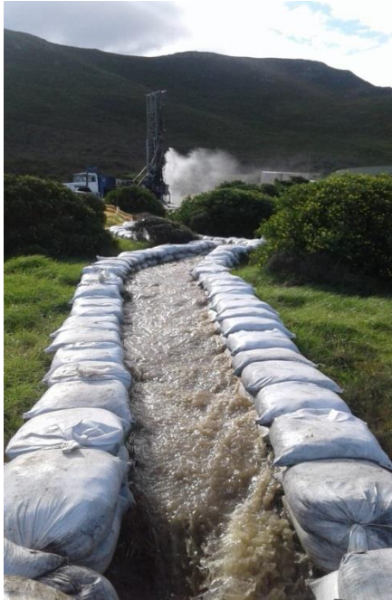
New borehole being drilled at the Gateway well field in Hermanus
