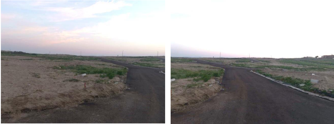
Blompark IRDP site, civil works completed
