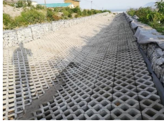
Hawston Housing project bulk storm water – completed
