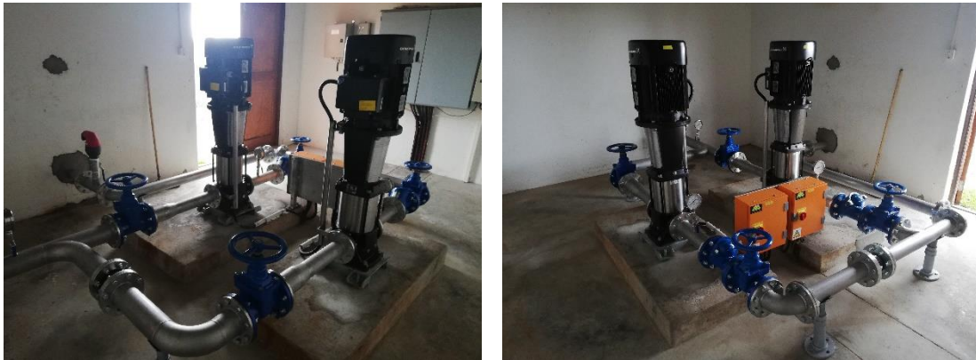
Hawston bulk water upgrade for Housing project – completed
