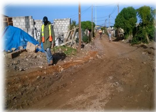
Roads under construction
