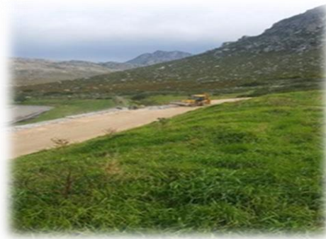
Phase 2- Under Construction
